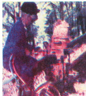
Fig 9 .11 Thermit process for joining railway tracks
