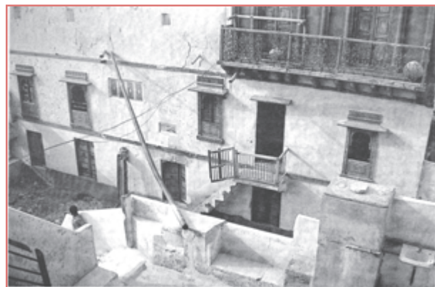
Rooftop harvesting was common across the towns and villages of the Thar. Rainwater that falls on the sloping roofs of houses is taken through a pipe into an underground tanka (circular holes in the ground), built in the main house or in the courtyard. The picture above shows water being taken from a neighbour's roof through a long pipe. Here the neighbour's rooftop has been used for collection of rainwater. The picture shows a hole through which rainwater flows down into an underground tanka .
